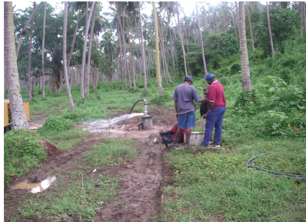
Bore Hole Drilling Santo
