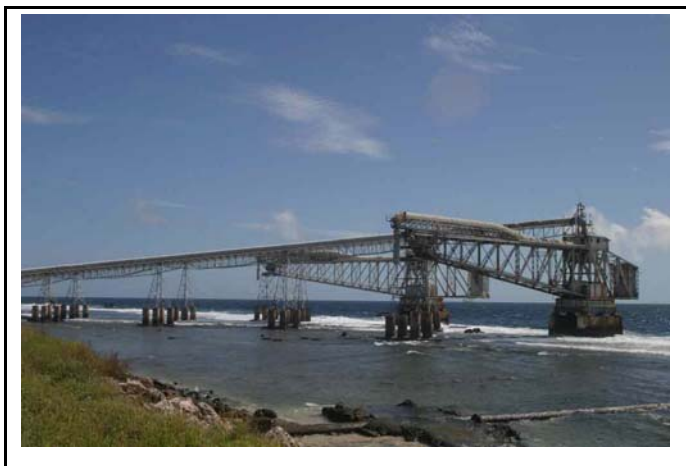
Figure 1.4 – Phosphate Cantilevers for Ship Loading
