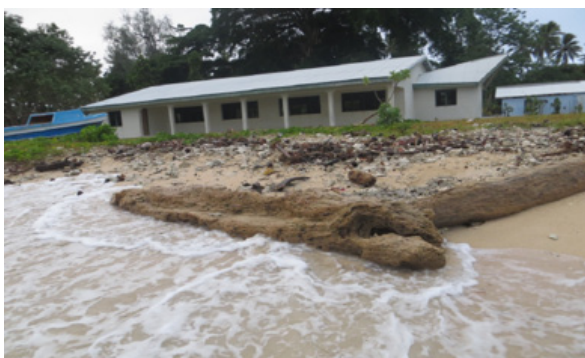
Figure 3.11: Coastal erosion threatening church building and households on Ahamb Island, Malekula. Credit: VCAP
