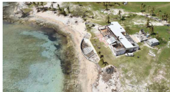
Figure 3.9: Aerial view of damaged hotel. Credit: Vanuatu TC Pam PDNA
