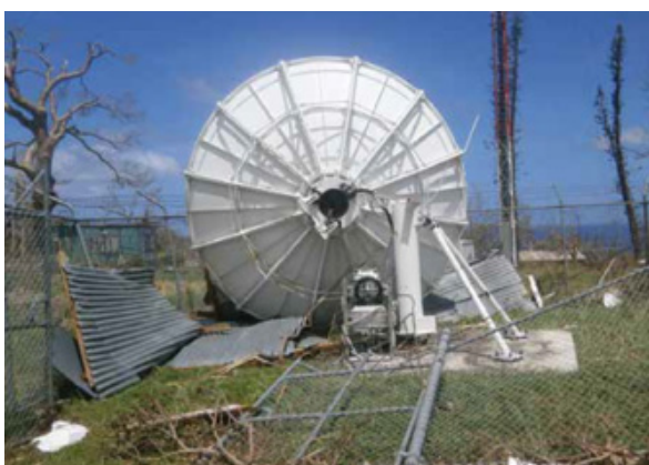
Figure 3.10: Destroyed satellite dish on Tanna island. Credit: Vanuatu TC Pam PDN
